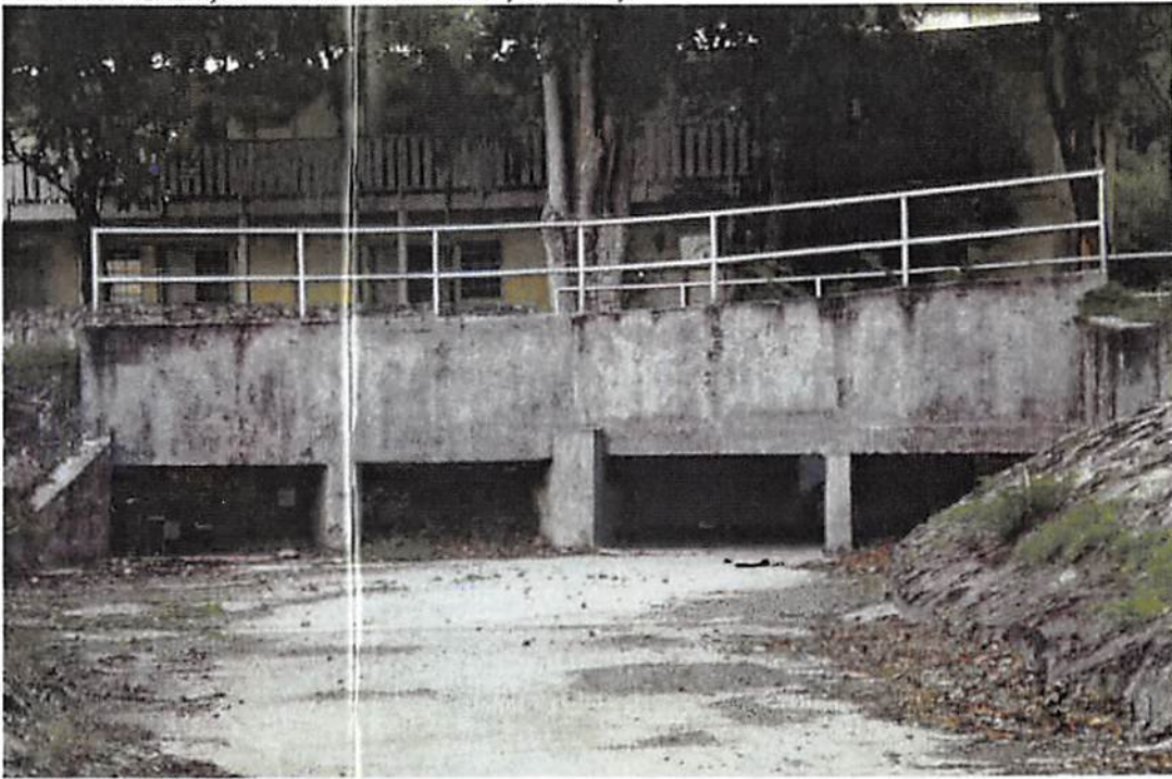
Figure 14: Sediment deposits in the Creek prevent boats from using the adjacent dock space
