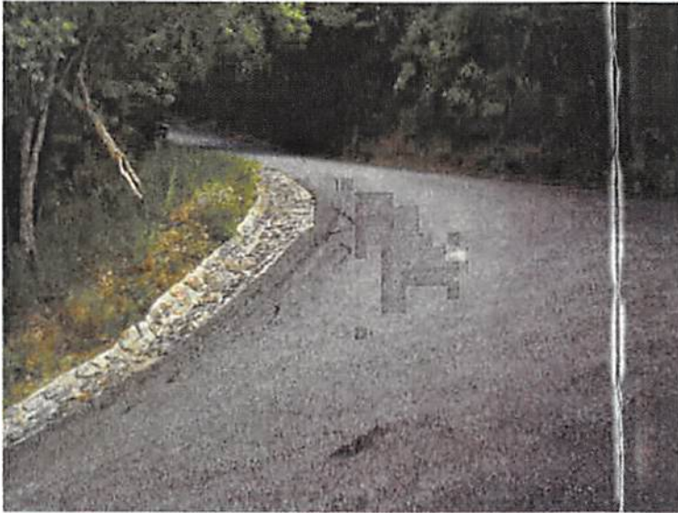
Figure 36: Trunk Bay Switchbacks
