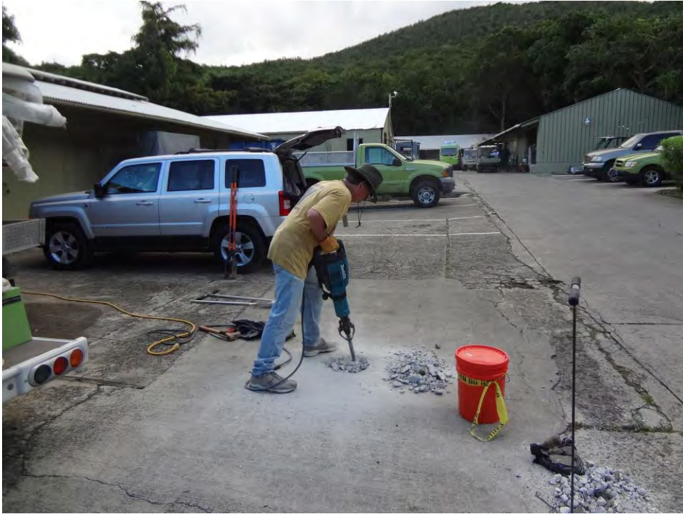
Former UST Location - Cutting Pavement for Borehole BH2
