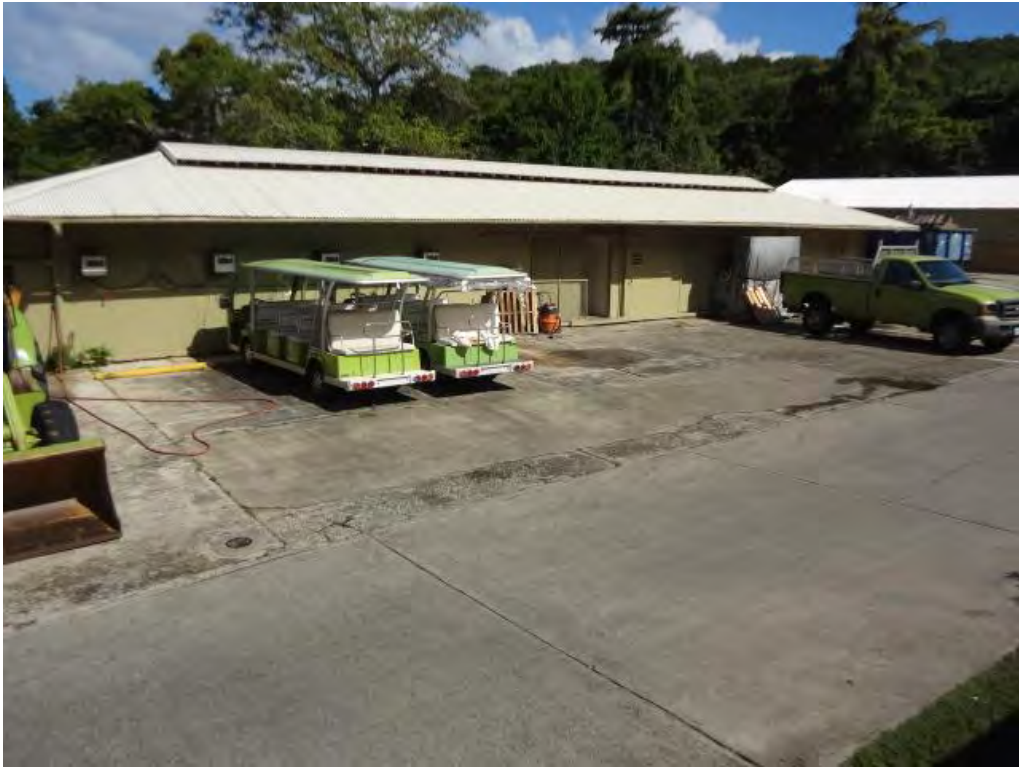
Former UST Location in Engineering Area
