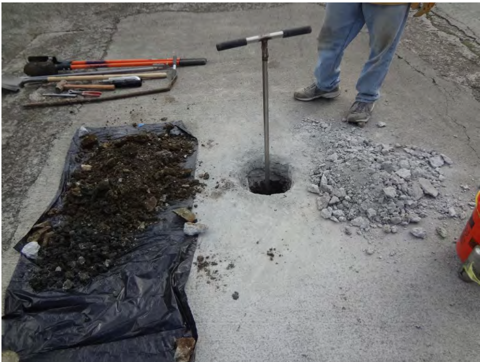
Former UST Location - Installing Borehole BH2
