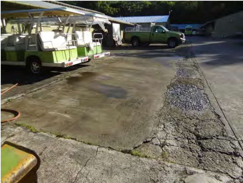
Concrete Pavement Patch at Former UST Location
