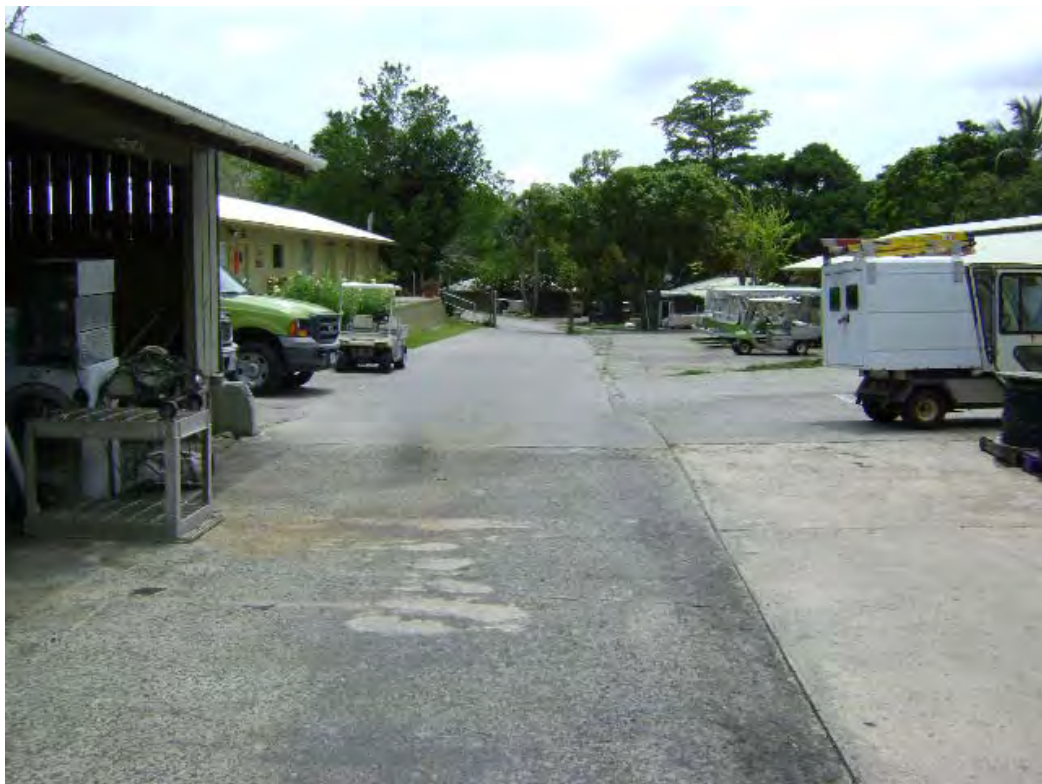
Engineering & Maintenance Area in Southeast Part of Subject Property
