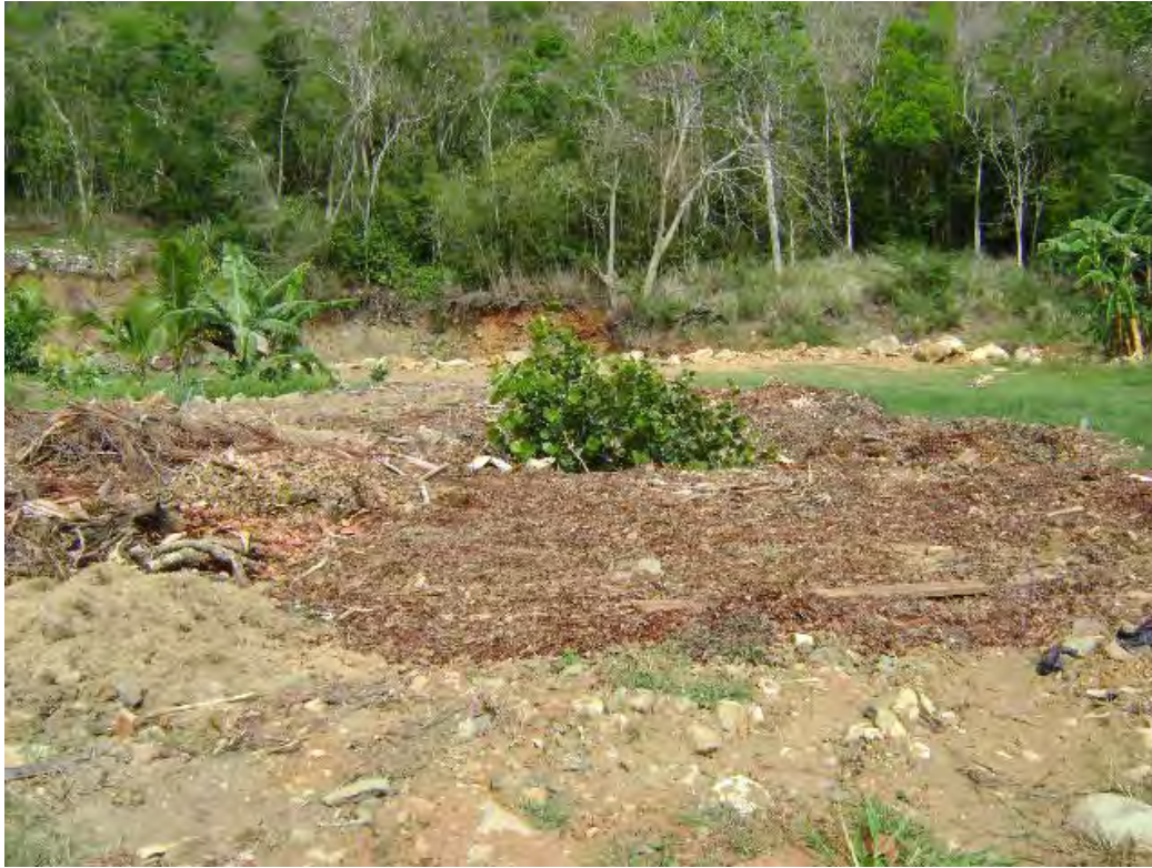
Debris Landfill Near Honeymoon Beach
