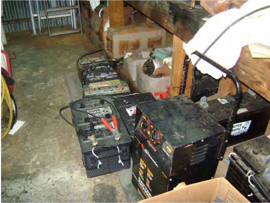
Batteries & Stains on Floor of West Building of Marina Facility
