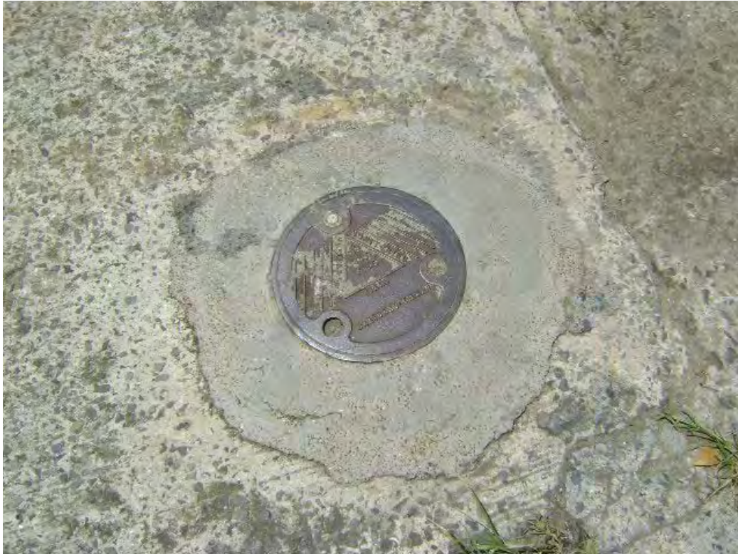
Monitoring Well in Pavement Near Diving Storage Building in Engineering & Maintenance Area
